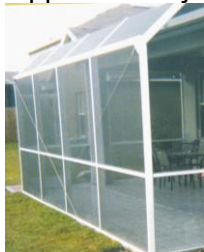
Example of approved design showing support cables
